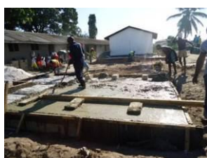
Construction of School latrines (foundation)
