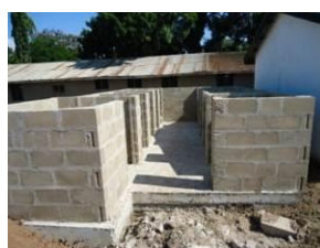
Construction of superstructure /latrine
